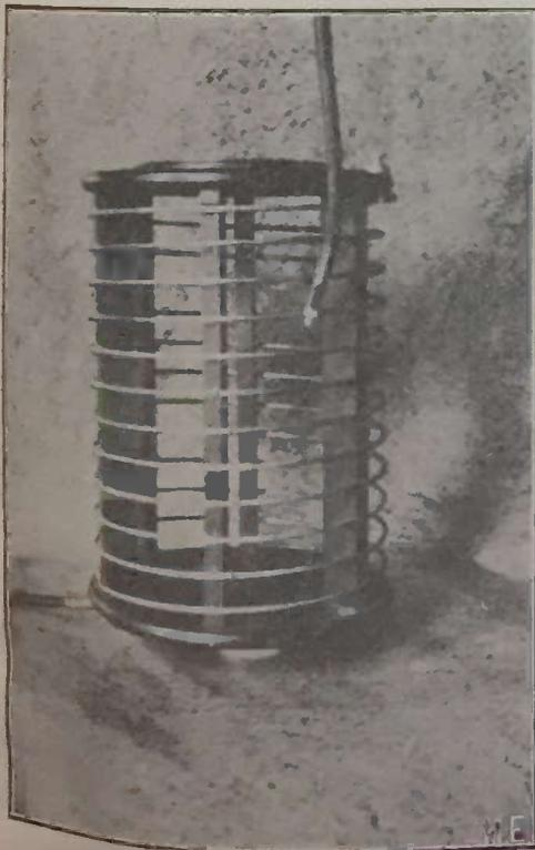
by any student in wireless signaling. The woodwork is of highly finished hard wood which should be well seasoned and dried. The convolutions are of solid aluminum wire and all the metal parts may be readily nicked and polished,
