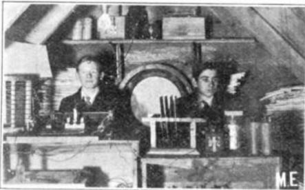
spark gap, and a glass plate condenser, having 8 x 10 inch plates.
