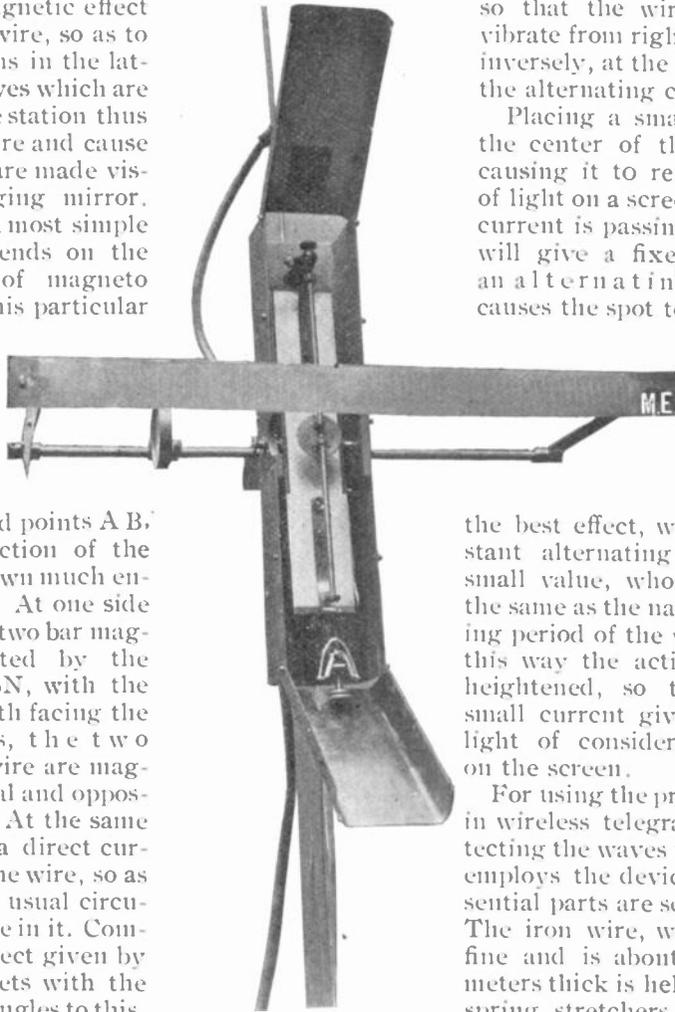
ror, and around the tubes is wrapped a spiral of insulated copper wire. This winding is in opposite directions in the upper and lower halves and the spiral is well insulated from the iron wire.
