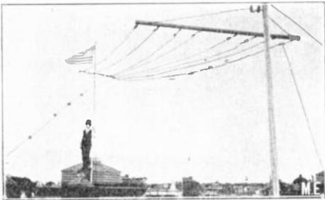
bare copper wires 50 feet long and one foot apart, strung from iron pipe masts on the roof. The iron pipe masts are made of 1¼ inch pipe, supported by guy wires. On each end of my aerial wires I have springs which always keep the wires tight and allow for shrinkage of the ropes in rainy weather.
