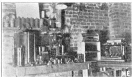
helix, heavy contact key and a S. P. switch conveniently placed at the right of the key for turning off the current. A porcelain base D. P. D. T. switch (shown in front of the coil) is used to throw the aerial and ground to either sending or receiving.
