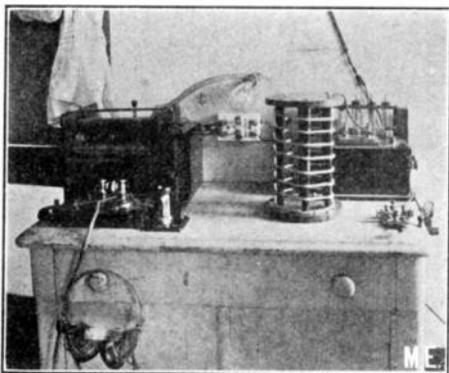
The receiving set consists of a large double slide tuner, E. I. Co.'s variable and fixed condensers, silicon and perikon detectors, with 2,000-ohm phones. A D. P. D. T. switch is used to throw in the sending or receiving apparatus. Nearly all of the instruments are of the E. I. Co.'s make.
