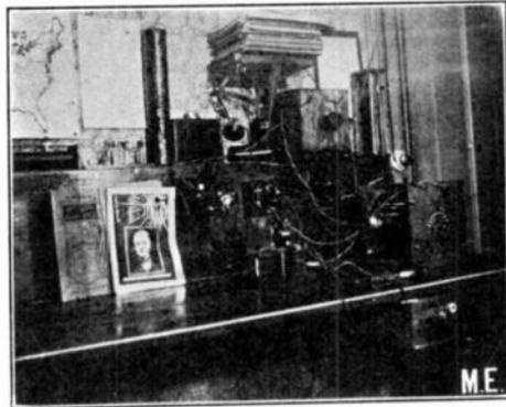
As can be seen in photo to the right of picture, upon a shelf by the door is a double slide tuning coil of 375 meters; next to this is a Variometer and a pair of 2,000-ohm E. I. Co. receivers; the big long coil standing next is the primary to my transformer and after this can be seen detector and potentiometer, and on the wall in order is a switch of my own construction of rotary type for receiving and sending. Snap switch for testing outfit and then silicon detector.
