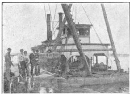
The cargo was valued at about \$45.00 per ton, and a loss of only about 10% resulted, the kegs being raised intact, and the nails uninjured except for slight rust, while a dredge if used would have broken the kegs open, and much of the cargo injured and lost. It will be noted that a great saving was realized by the use of the lifting electro-magnet instead of a dredge, which would have been difficult to operate, as the kegs of nails were raised from a depth of 70 feet.
