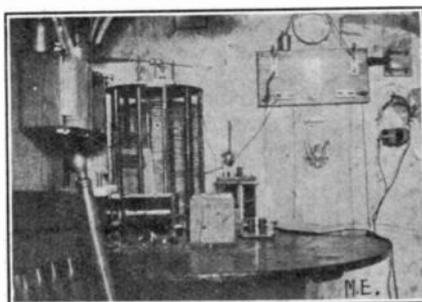
ers (under table and operated from above), electrolytic and silicon detectors with 3,000-ohm phones.
