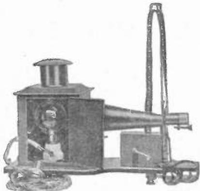
ACETYLENE MOVING PICTURE MACHINE.
