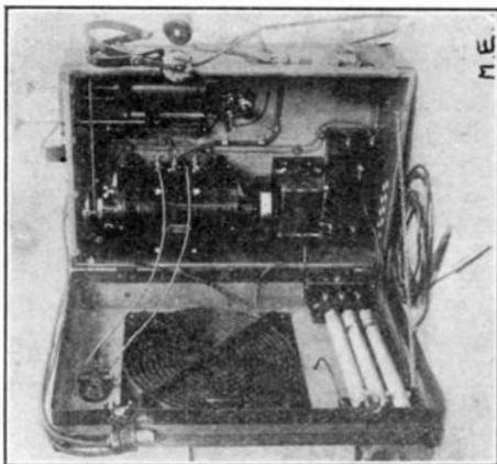
and enhance the sending power. The complete outfit can easily be carried by one man.
