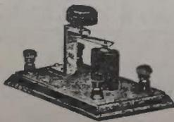
If you wish a fine relay, having extraordinary sensitivity micrometer adjustment, use the Gernsback relay, on account of its novel design and its great simplicity. It is by far the cheapest relay on the market to day. It was constructed mainly for wireless work, but, can of course be used for all other purposes where an extremely sensitive relay with fine adjustment is needed.
