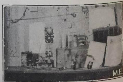
tors, one silicon, the other peroxide of lead, 1 coherer and decoherer (seen on the wall), 1 variable condenser, 1 fixed condenser (not seen in picture), 1 D. P. D. T. switch to receive or to send, batteries to work with the coherer and decoherer, and 2,000 ohm head set. All
