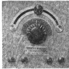
A tuning transformer possessing greatly increased range and selectivity: all adjustments are actuated by the rotation of thumb nuts upon the face of the instrument.
