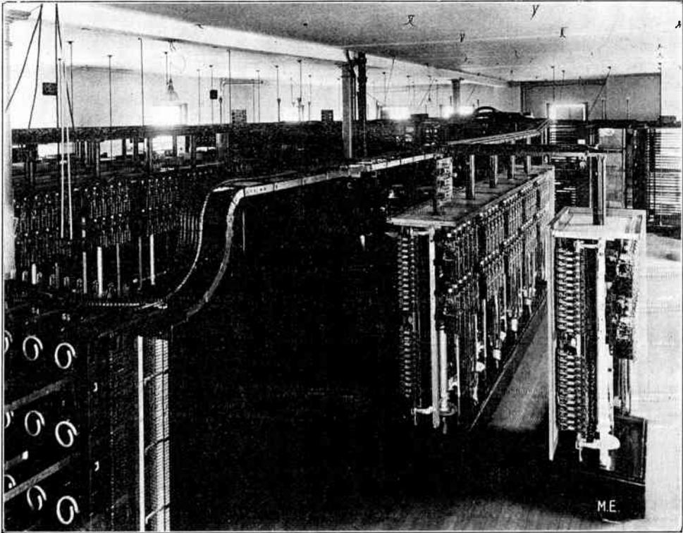
FIG. 8.—AUTOMATIC TELEPHONE EXCHANGE AT HURON, SOUTH DAKOTA "NOT A GIRL IN SIGHT"
