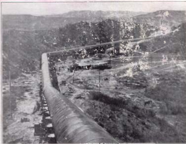
A NINE-MILE SIPHON—PART OF LOS ANGELES' HYDROELECTRIC SYSTEM
