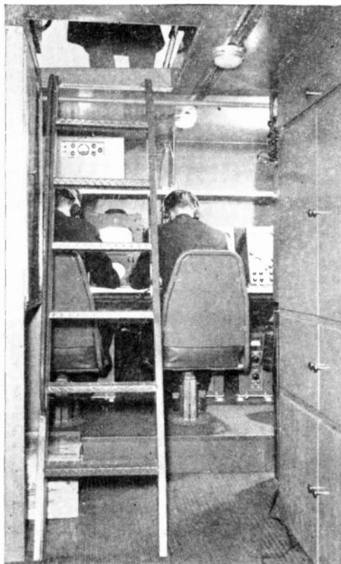
Inside a mobile TV unit. Ladder provides access to the roof hatch
