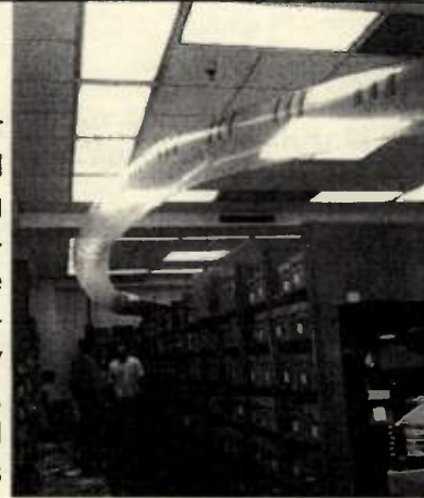
The Archives' ceiling was snaked with dehumidification equipment from Munters Moisture Control Services
