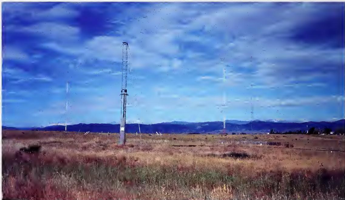
Figure 3.4. 15 MHz WWV Antenna (WWVB Towers in Background)
