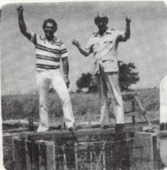
Ron Dryden and Paul stand on the footing to the great TV tower that will beam the Gospel all over Oklahoma!
