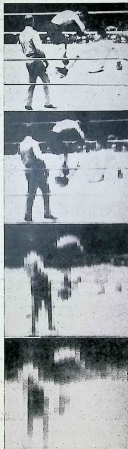
Fig. 1.—Something for the future to aim at. To transmit such pictures at the minimum required rate of 16 per second will take about 8,000,000 pulses or 4,000,000 cycles per second. This is about 400 broadcasting channels or everything from 545 meters down to 66 meters! The pictures have 250,000 "elements" each. The amplifiers must handle all frequencies from 16 cycles to 4,000,000!
