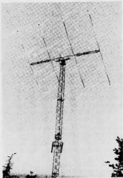
Fig. 3—This 2-meter EME array at I2OD1 is built from 16 long-boom Yagis. Arrays like this are great to have, but smaller antennas can work, too.
