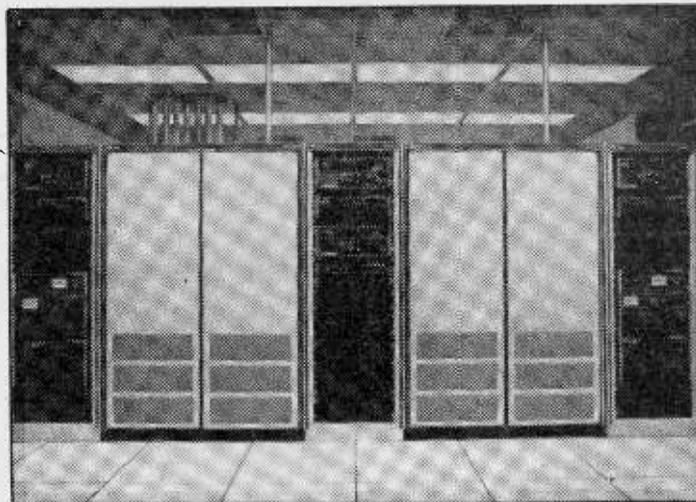
Collins HF-80 series HF radio equipment is front stage center in the Comm Central Equipment Room.
