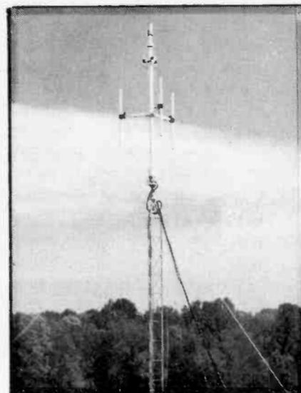
The interferometer antenna system.
