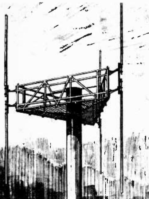
Los Angeles cellular telephone, call sign KNKA 351, is typical of the non-wireline bandplan. Base transmit conversations may be heard every 30 kilohertz from 875.580-876.090 MHz. Mobile transmissions will be exactly 45 megahertz lower.
