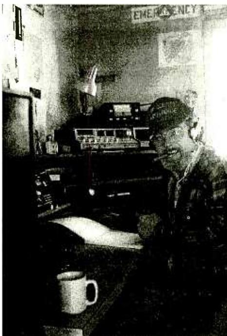
*Ed Barnat, Tri-County 44, fulfills CB's potential for mutual aid by standing the afternoon shift of RoadWatch. The boom microphone on the headset is for on-the-air traffic broadcasting. The audio output from eight scanners are brought into a mixer and into the headset.*
