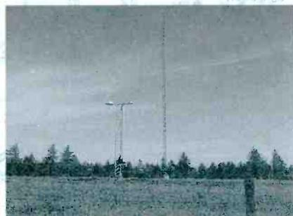
*GWEN Tower and GPS antennas at Appleton Washington, used to demonstrate NDGPS concept.*
