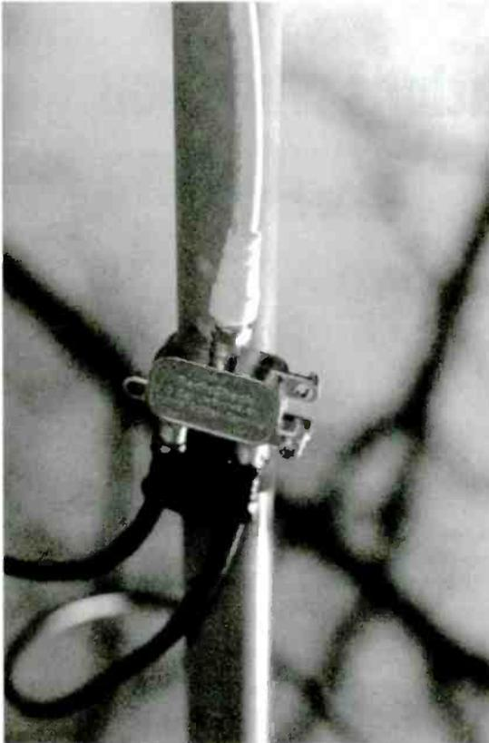
*Attach feed line from receiver to the bi-directional coupler. Cover all "F" connectors with silicon or Coax-Seal® and lash the connector to the mast. When installing the feed line into the house, make a drip loop to prevent rain leaking into the house.*
