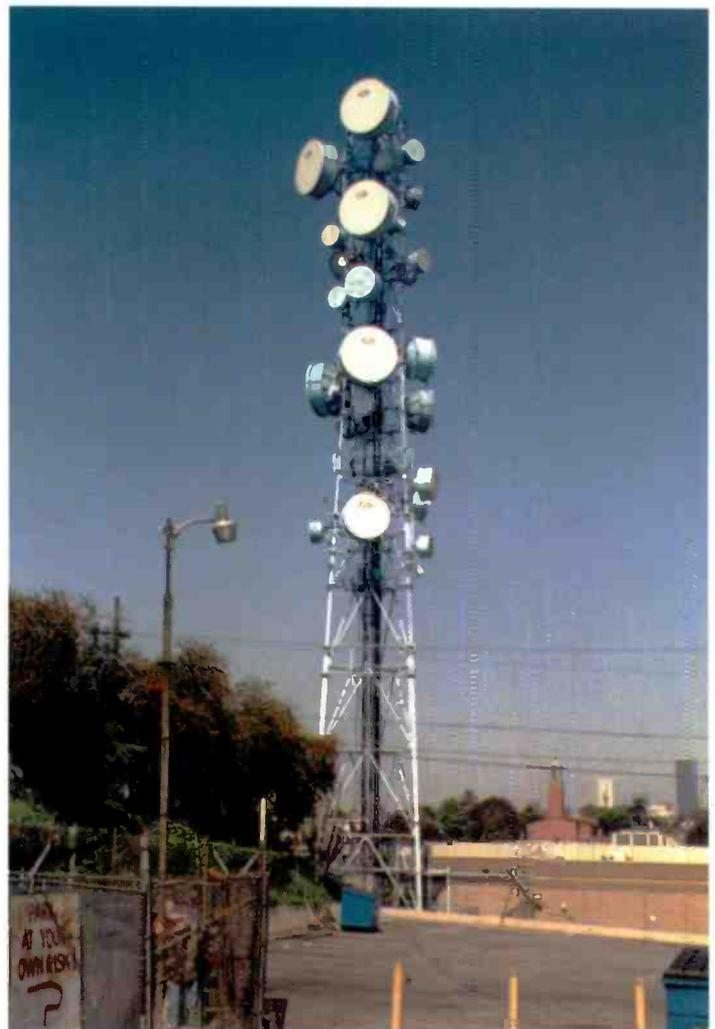
*While it would be tempting to say this is an all-weather test rig for kettledrums, in fact it's a microwave hub for a telephone network. The purpose is to combine thousands of telephone calls by multiplexing them on a microwave radio link rather than to have to provide hardwire lines for them. (Photo submitted by Al Shack, Simi Valley, CA)*
