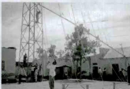
*Setting up Radio Galkayco's log periodic antenna in 1994 and how it looked when it was completed*
