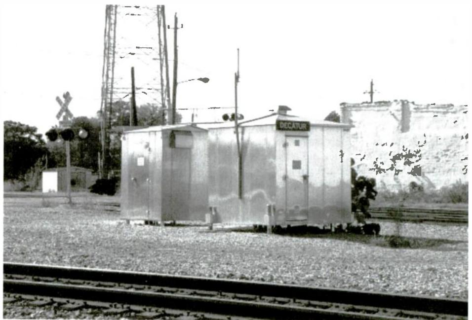
*These prefabricated sheds, located in Decatur, Alabama, house electronics and radio equipment for controlling signals and switches.*
