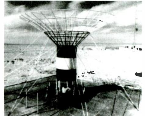
Example of a Cross Field Antenna similar to one which Music Mann 279 plans to use. The 9 meters high model is currently radiating 100 kilowatts from a site at Barnis is Southern Egypt, on 603 kilohertz (approx 495 meters Mediumwave)
