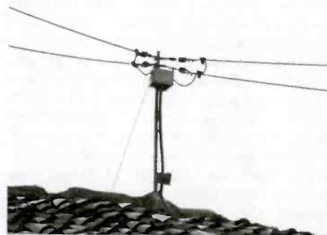
A close-up of antenna feeder (now only 2-band: 75 and 41 m)
