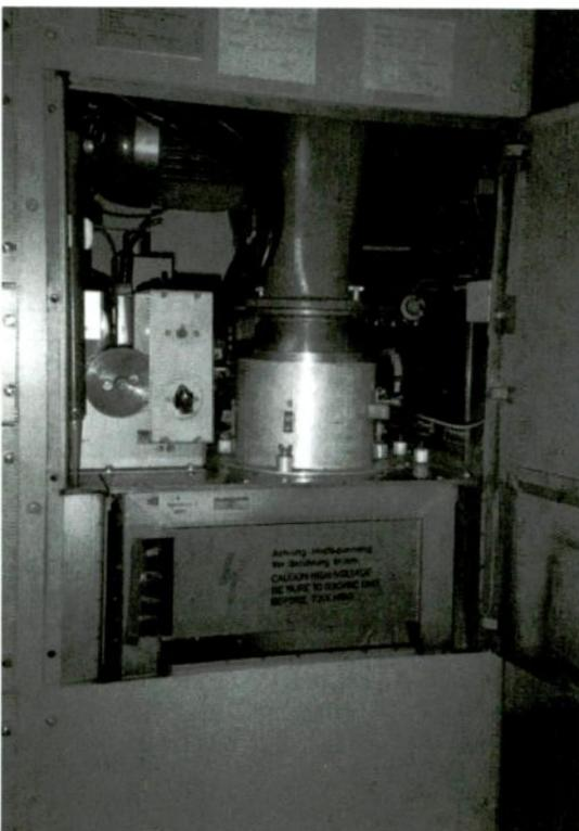
*A close-up of the transmitter final section*
