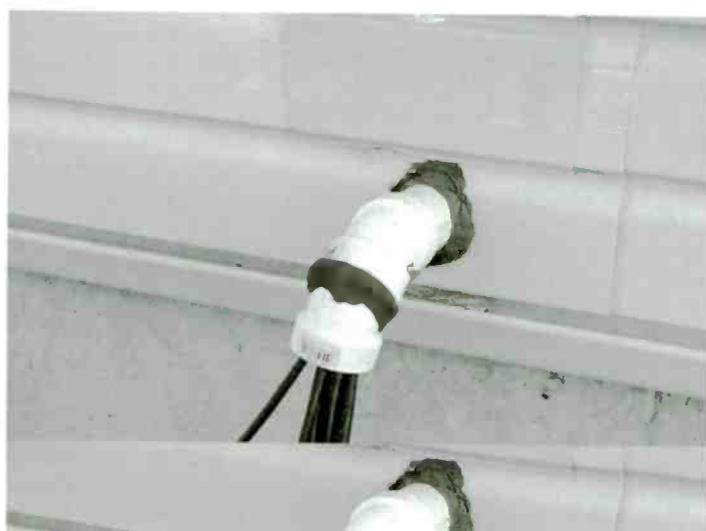
Denis Dandeneau's solution to the antenna lead-in problem. Easy to find and work with, PVC pipe is fitted through a hole cut with a low cost 2" hole saw that fits on your drill. (Courtesy Denis Dandeneau)
