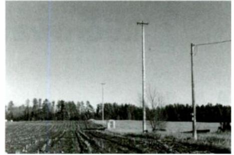
Mike Leahan (WI) sent this photo of SLY (344 kHz) near Hayward, WI. Although not visible here, the antenna consists of two parallel wires strung between the cross-arm utility poles. The shed houses the beacon transmitter.
