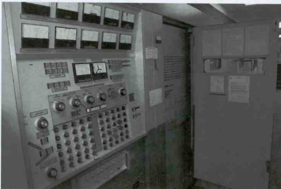
Transmitter four's control panel, with the door open for frequency changes
