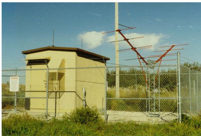
“V” shaped antennas at many longwave sites are for a separate 75 MHz marker beacon. This one is at LH/334 kHz, Bloomington, IL.
