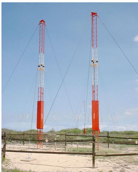
**WWVH 15 MHz antenna array: Two half-wave vertical dipoles separated by a quarter-wave length and driven 90 degrees out of phase. (Courtesy: NIST)**
