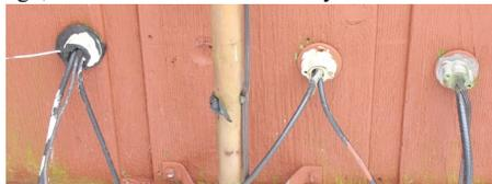
*Not so pretty solution. Using Radio Shack clear plastic feed through tubes (no longer available) an assortment of cable of various dimensions make it into the house, note the Coax-Seal that stops critters and rain. (Courtesy: Author)*
