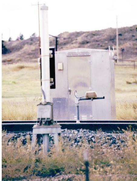
*Wayside scanning equipment for reading RF tags on railcars and locomotives. The small box on the inverted L-shaped arm is the transmitter. The larger antenna on the vertical post reads the signals that are returned. The angle of the photo makes it look like the transmitter unit is between the rails. It is not.*
