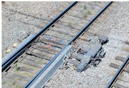
*Power switch mechanism. This power switch is part of a cross-over, which in turn, is part of the Boylan Interlocking in Raleigh, N.C. The covered sheet metal channels outside the rails are part of the switch heater, which during precipitation in below-freezing weather, keeps the switch from freezing up or being blocked by ice or snow.*
