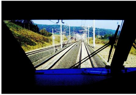
*View from the engine of a German ICE high-speed train doing more than 150 miles per hour. This photo was made back in 1991! Note the continuous antenna running between the rails that is used to communicate data and instructions between the dispatching center and the train.*
