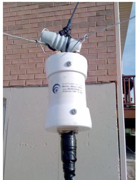
**Fig 2: The 4:1 Balun and strain insulator.**
