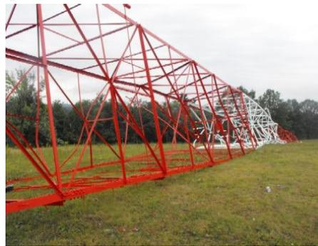
One of three 400' WWVA towers on the ground after wind storm (Courtesy: WWVA-AM)
