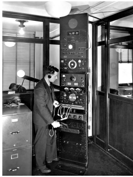
*W8XWJ shortwave receiving and monitoring station 1-24-1936. Equipment includes (top to bottom) a Western Electric monitor amplifier and speaker; oscilloscope modulation monitor; General Radio frequency meter; National HRO receiver; Western Electric meter panel; Hallicrafters SX-10 Ultra Skyrider receiver; audio mixer and switch panel. The operator is not identified. (From the Detroit News Archives)*
