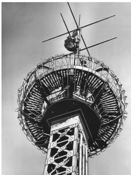
W45D FM antenna 1-27-1942. The two bay turnstile antenna of W45D above the beacon on top of the Penobscot Building. The workman is Ted Ryerse. (From the *Detroit News* Archives)
