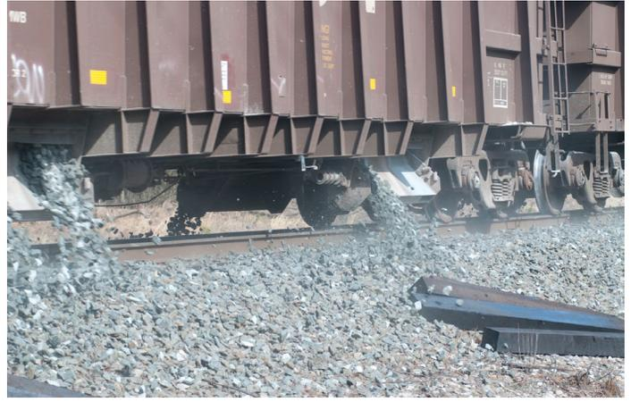
*This car in the GPS-controlled Herzog ballast train has just passed a grade crossing and the discharge gates are in the process of opening and resuming the ballast dumping process. The train is dumping ballast on the outsides of both rails but not between the rails.*
