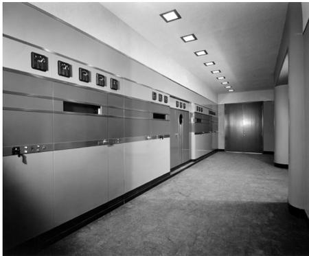
*KWID's new 100 kW General Electric transmitter is shown installed and ready to turn on; February, 1942. (Photo courtesy of FEBC International)*
