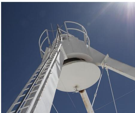
Here is the highest point on the dish, the secondary reflector. 'Signals,' or noise, from space are reflected off of the dish back up to the steerable reflector above the main dish and back down into one of several selected horn 'antennas' that are located below the surface of the dish. It's a similar scheme as the Schmidt-Cassegrain optical scope configuration. No, we didn't climb up the ladder - Dave said that takes a course how to use the safety cable.
