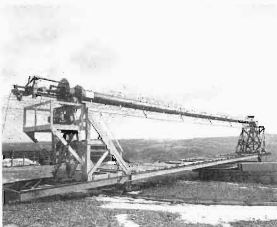
Fig. 47. Three bay, VHF high band Helical Antenna (GE Photograph).
