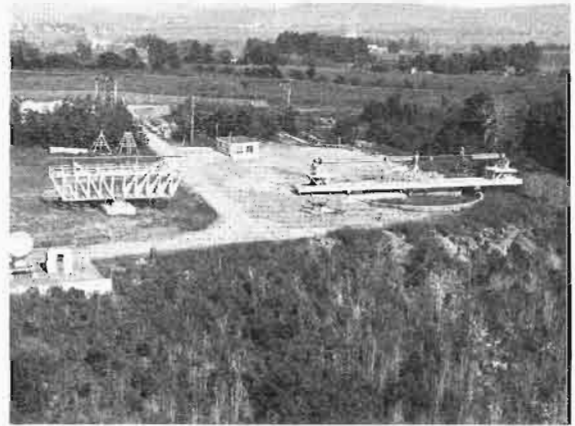
Fig. 71. Turnstables at Cazenovia Test Site (GE Photograph).
