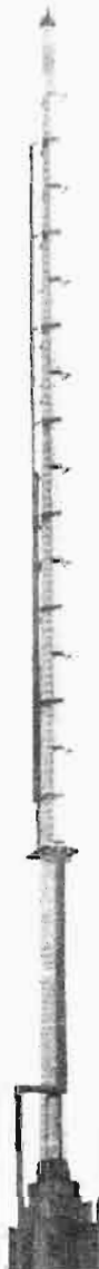
Fig. 69. A 16 element directional long-slot UHF antenna at Station WXTV, New York, N.Y. (Alford Photograph).
