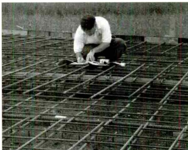
Paul Mucci of Civil Engineering firm Aerial Spectrum checks foundation rebar placement against the drawings before the transmitter building foundation is poured.
