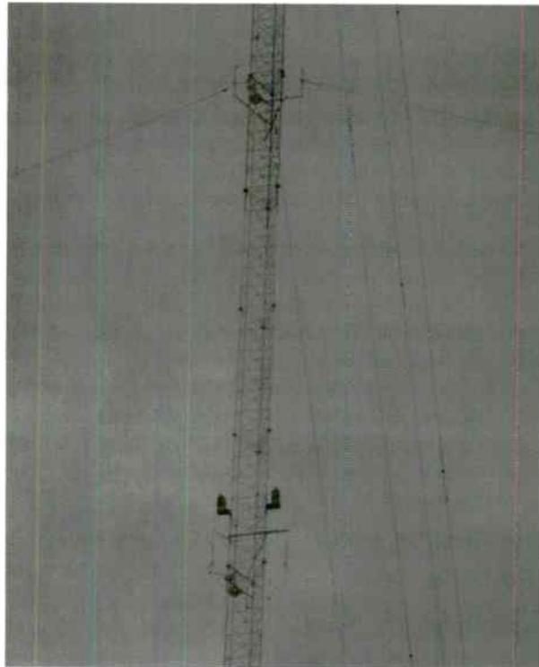
The detuning skirts can be seen, one below the center beacons, one just above where the orange section starts above the beacons. You can also see the capacitor boxes.
