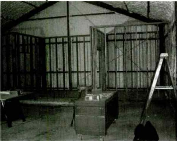
Insulation has been blown in and the framing is in for the bathroom and studio areas.
