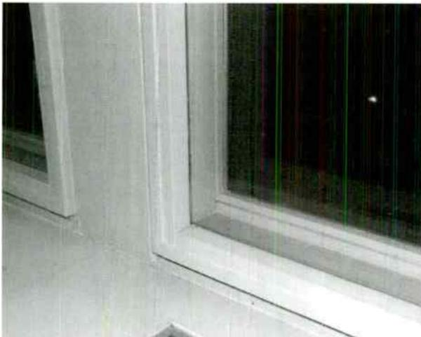
The inside window in front of the outside window. This piece of plate glass reduced noise from outside by greater than 60dB.
