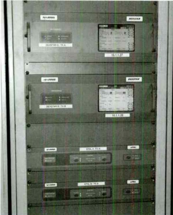
The HD rack sits between the transmitters. Each transmitter has its own HD exciter.
