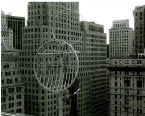
The STL antenna, AM receive loop, and DirecTV dish on the roof of 111 Broadway. Note that the Mark grid dish is painted the same color as the penthouse. The AM loop antenna should be pointing at the camera, but offers no signal in that direction.
