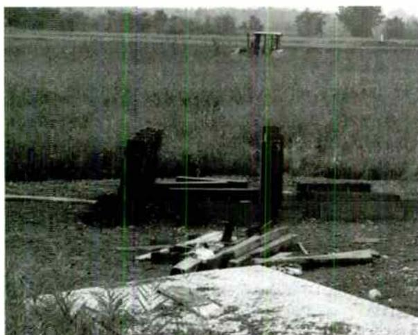
A guy anchor location. Note the angled piles on the left, toward the direction of guy wire pull.
