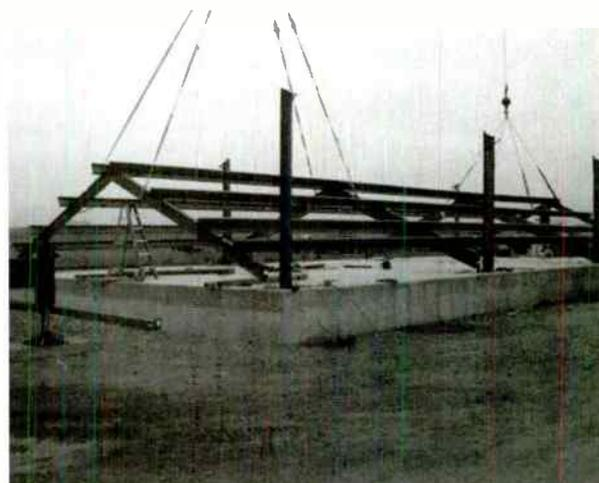
The roof trusses ready to be hoisted into place.
