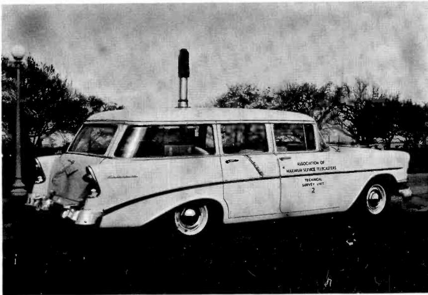
Figure 1 - MST Mobile Survey Unit No. 2. The hydraulic mast is shown in the retracted position for traveling.
