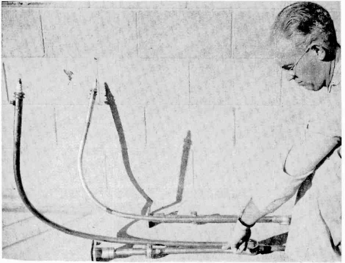
The matching harness is made from Andrew type S-450 7/8" co-ax. This line is available from the factory with dipole end terminals, using gas tight construction. The junction box ends of these lines may be cut and soldered on the job, depending on local measurements.
