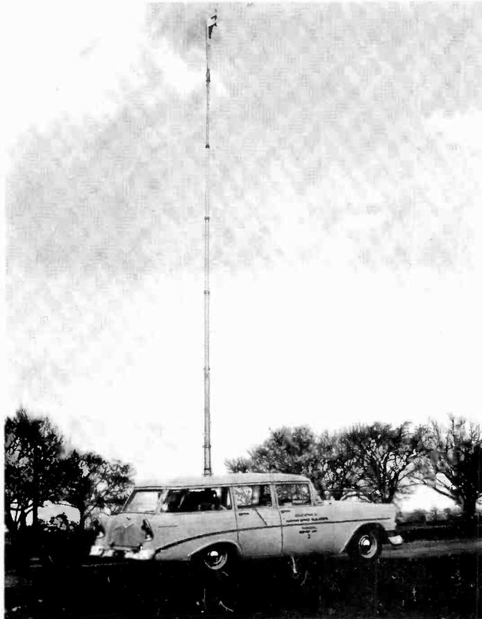
Figure 2 - Mobile unit with mast extended to 30-foot height. A UHF antenna is mounted on the mast.
