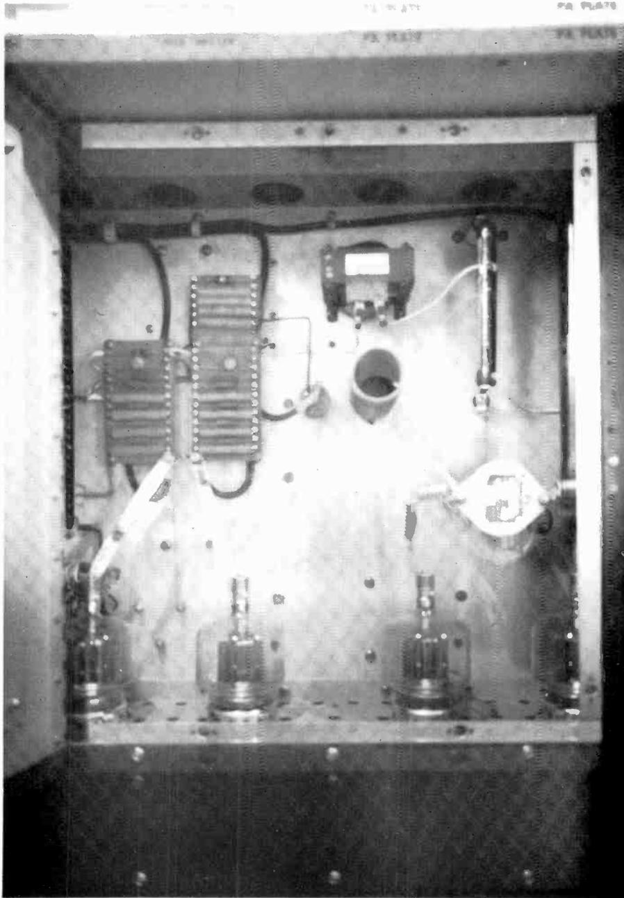
FIG. #4 - TUBES IN 1KW TRANSMITTER IN NORMAL
