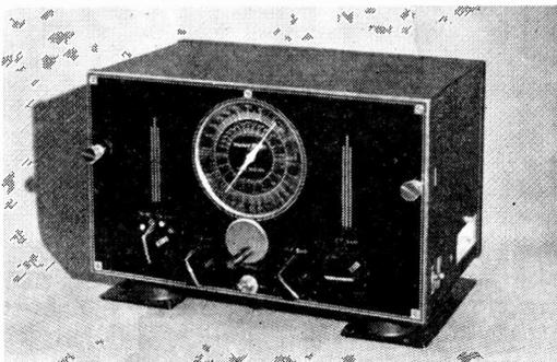
The new 20A aviation Radio receiver with controls mounted on front panel for direct operation when unit is installed within easy reach of pilot.
