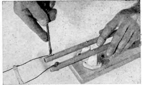
The half-wave open-wire antenna is constructed from two 5' lengths of 1/2" aluminum tubing. Make a smooth right-angle bend at the midpoint of each tube to form the Q-matching transformer.
