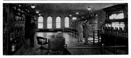
View of Main Operating Room, WENR, Chicago. Along the right wall are the high-power Radio frequency amplifiers, and the modulators, equipped with 20-kilowatt water-cooled tubes. On the left are the power supply panel, and the intermediate Radio frequency amplifier.
