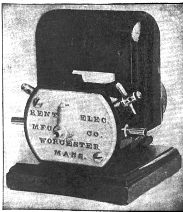
DYNAMO FOR GAS ENGINE IGNITION.
