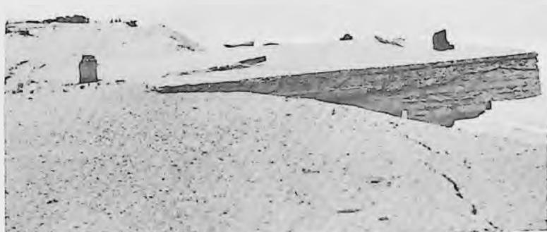
BASE OF THE OUTER TOWERS IN 1945. DUE TO THE EROSION, IT WAS NECESSARY TO CUT THE TOWER DOWN IN 1920. TODAY THE CLIFF HAS BEEN CUT BACK TO THE TRANSMITTER HOUSE FLOOR, WHICH WAS THE CENTER OF THE FOUR TOWERS.
