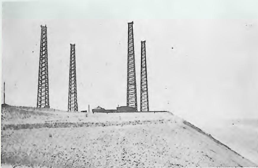
THE FOUR TOWERS WERE THEN ERECTED AT THE EDGE OF THE CLIFF. IN 1902 THEY WERE NOT AS CLOSE TO THE EDGE AS HERE IN 1917. THE OCEAN HAD BEEN ERODING THE SHORE IN THE MEANTIME. A LONELY PLACE WITH NO COMMERCIAL POWER REQUIRING THE USE OF OIL ENGINES AS PRIME MOVERS.
