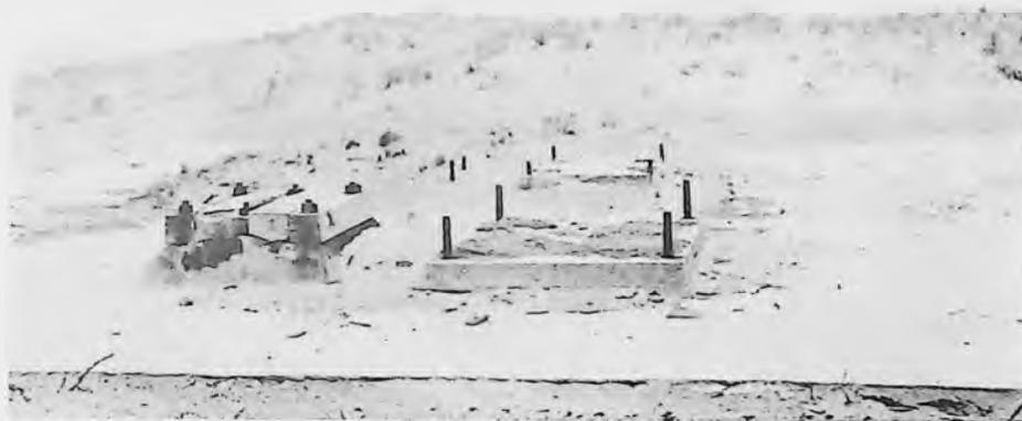
1941 - FLOOR OF THE TRANSMITTING HOUSE. FRONT LEFT IS THE MOUNTING OF THE FAMOUS ROTARY SPARK GAP, AND TO THE RIGHT, THE STUDS FOR THE ROTARY MOROR. REAR LEFT SAT THE BIG GLASS PLATE CONDENSERS AND REAR RIGHT VERTICALLY MOUNTED HELIX OR WHAT MARCONI WOULD PROBABLY CALL A JIGGER.
