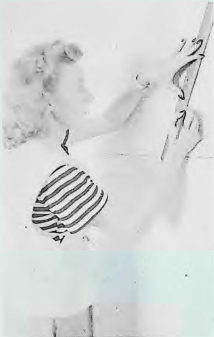
RID GIRL TAKING A HIGH FREQUENCY BEARING WITH ADCOCK D.F. AND PLOTTING BEARING.
