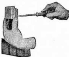
FIG. 4,132.—*How to assemble an air circuit breaker 3.* Method of attaching stationary carbon burning tip to bracket.
