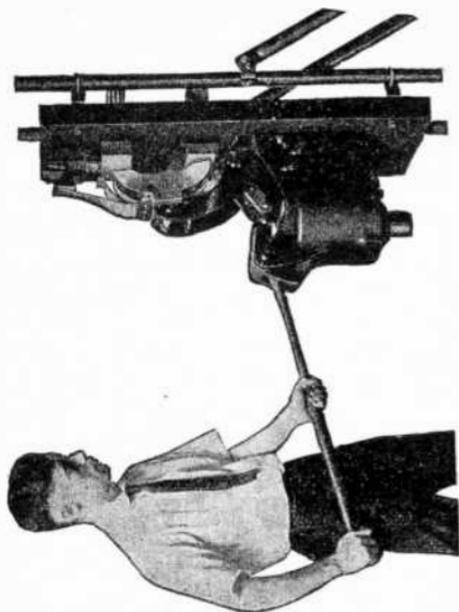
FIG. 4,189.—How to assemble an air circuit breaker 28. Closing solenoid operated air circuit breaker with hand lever.
