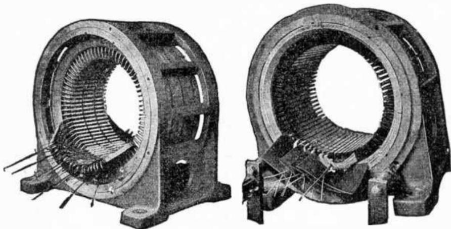
FIGS. 2,787 and 2,788.—General Electric slip ring motor construction 1. Partially wound fields showing exposed laminations, oiled paper and linen slot insulation, form wound coils wrapped with "assembly" or (sacrifice) tape which affords protection while installing, and a perfect fit in the slots.
