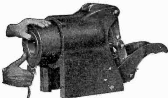
FIG. 4,168.—How to assemble an air circuit breaker 17. Inserting the operating coil in the solenoid magnet frame.
