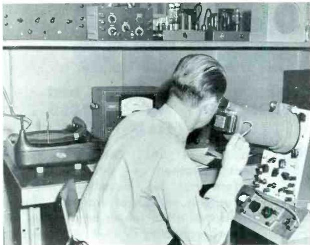
A picture of some of the equipment used in connection with measurements and waveforms appearing in this article. The instrument in use is an oscilloscope fitted with a scope camera.
