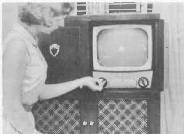
Figure 4. Typical Spot on Television Screen After Receiver is Switched off.
